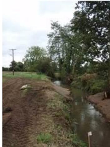
After: Berms on each side give a more sinuous channel, the gravel bed and varying depths will reduce Bur-reed growth
