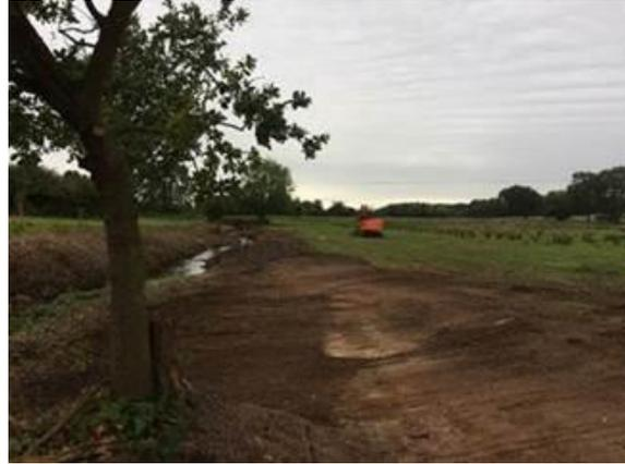
After: more natural bank profile, which allows river to spill out with a shallow fast flowing section during normal flows.
